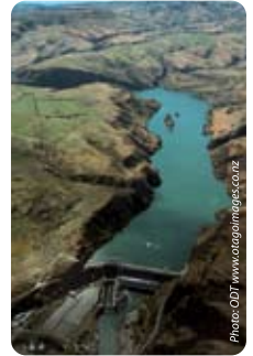
Aerial view of the Roxburgh dam and Lake Roxburgh
