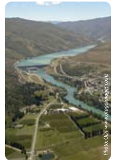
Aerial view of the Clyde dam with the township of Clyde to the right
