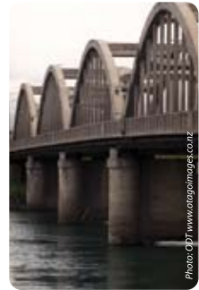
The Balclutha bridge, with its distinctive bowstring design
